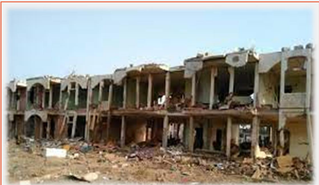
The destruction caused by the aggression targeting the housing of the Mokha station employees
